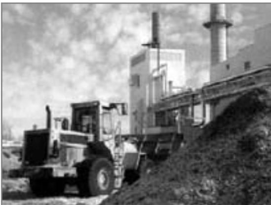
*A power plant in the US, which produces electricity through gasification of wood chips*
